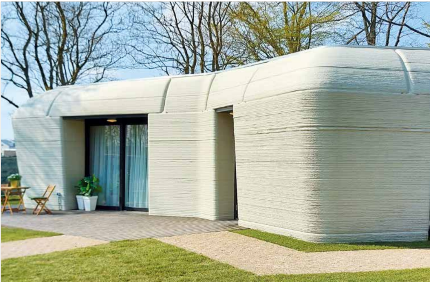
3D geprinte woning in Eindhoven (Project Milestone).
